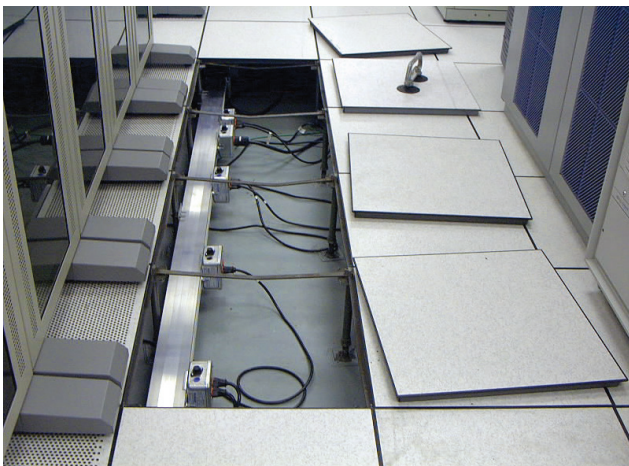
A clean, organized power busway system simplifies power distribution and can lower HVAC costs.
