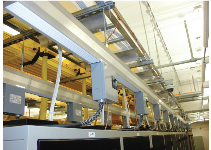
Power can be accessed at any location along the busway system, eliminating the need for power boards, long runs of wire and expensive installation costs.
