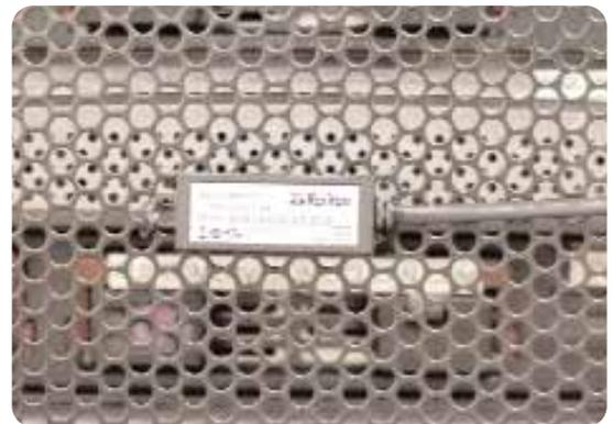
An example of a temperature sensor mounted at the cold air inlet of a server rack. Sensor is connected to an intelligent PDU (not shown).
